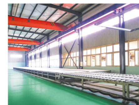
后输送线 Behind conveyor plant
